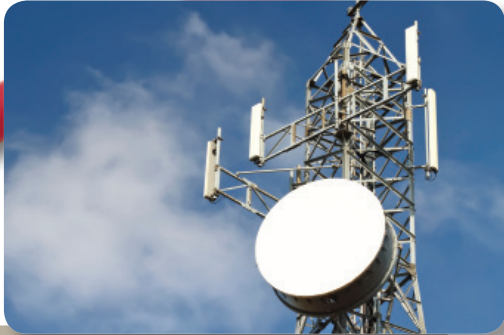
WIRELESS CELL TOWERS
